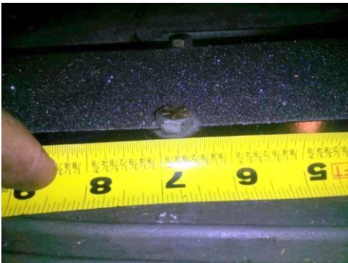
Position bolt 6 3/4" in from right side of bracket
